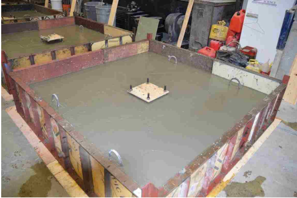
Figure 3-11: Completed Footing
