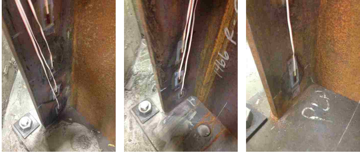
Figure 3-31: Installed Strain Gages
