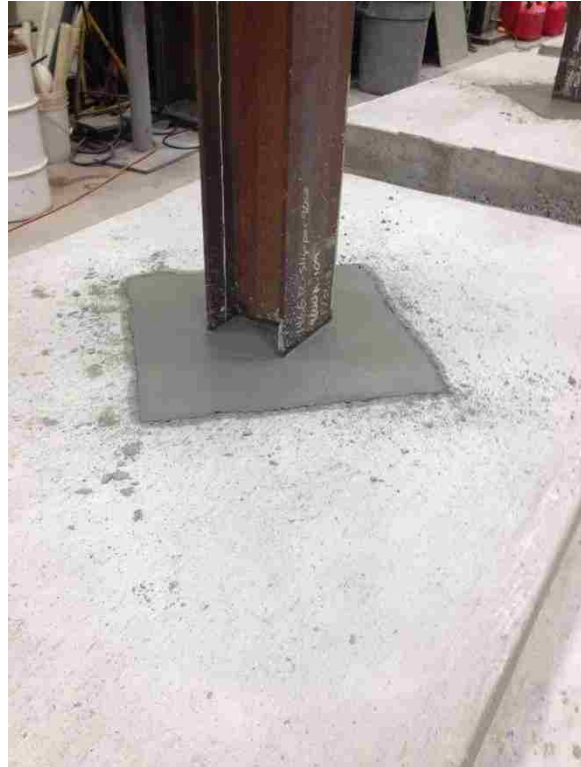
Figure 3-19: Column After Filling the Block-out
