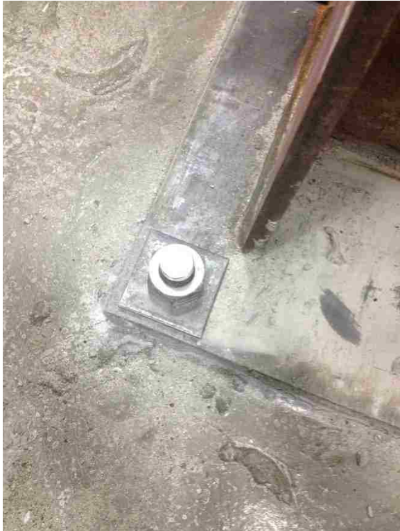
Figure 3-18: Bolt and Washer Installed on Grouted Column
