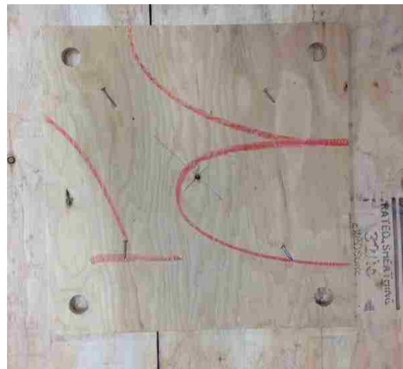
Figure 3-9: Anchor Rod Guide
