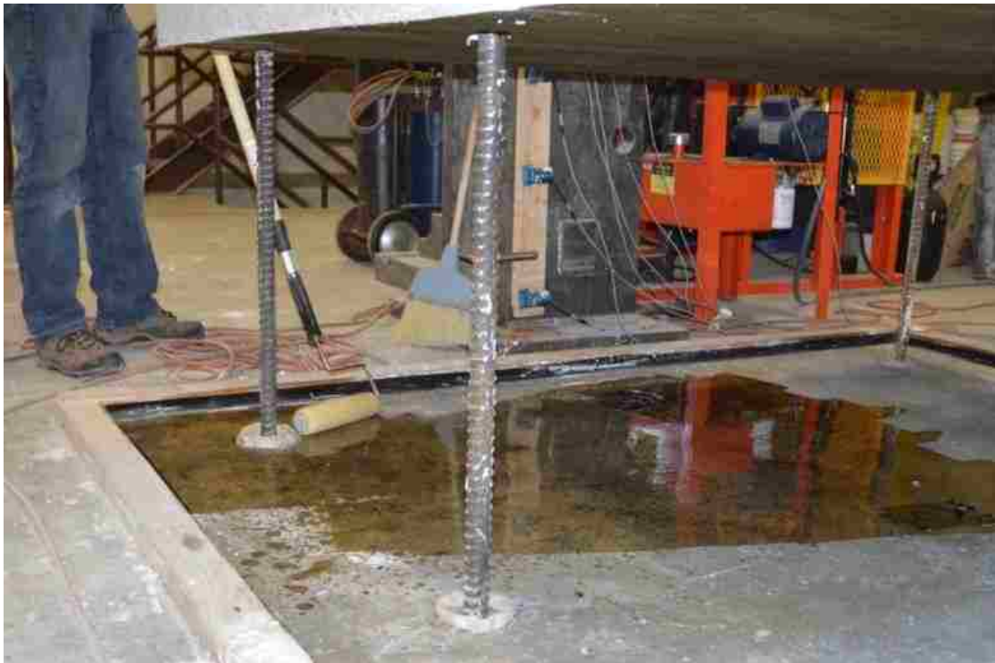
Figure 3-23: Applying Form Release to Lab Floor
