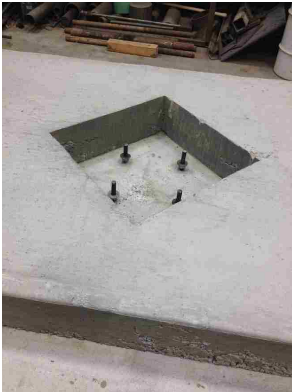
Figure 3-16: Leveling Nuts and Washers
