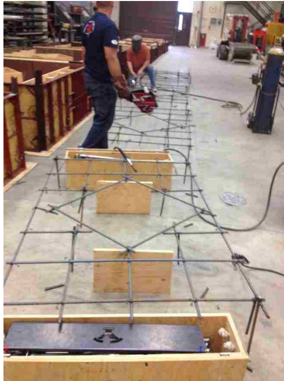
Figure 3-13: Welding on Rebar Chairs
