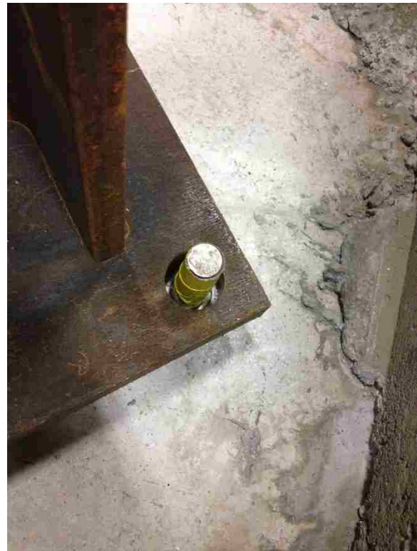
Figure 3-17: Column on Leveling Nuts and Washers
