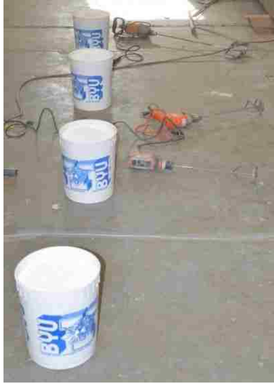
Figure 3-24: HYDROCAL Mix Preparation
