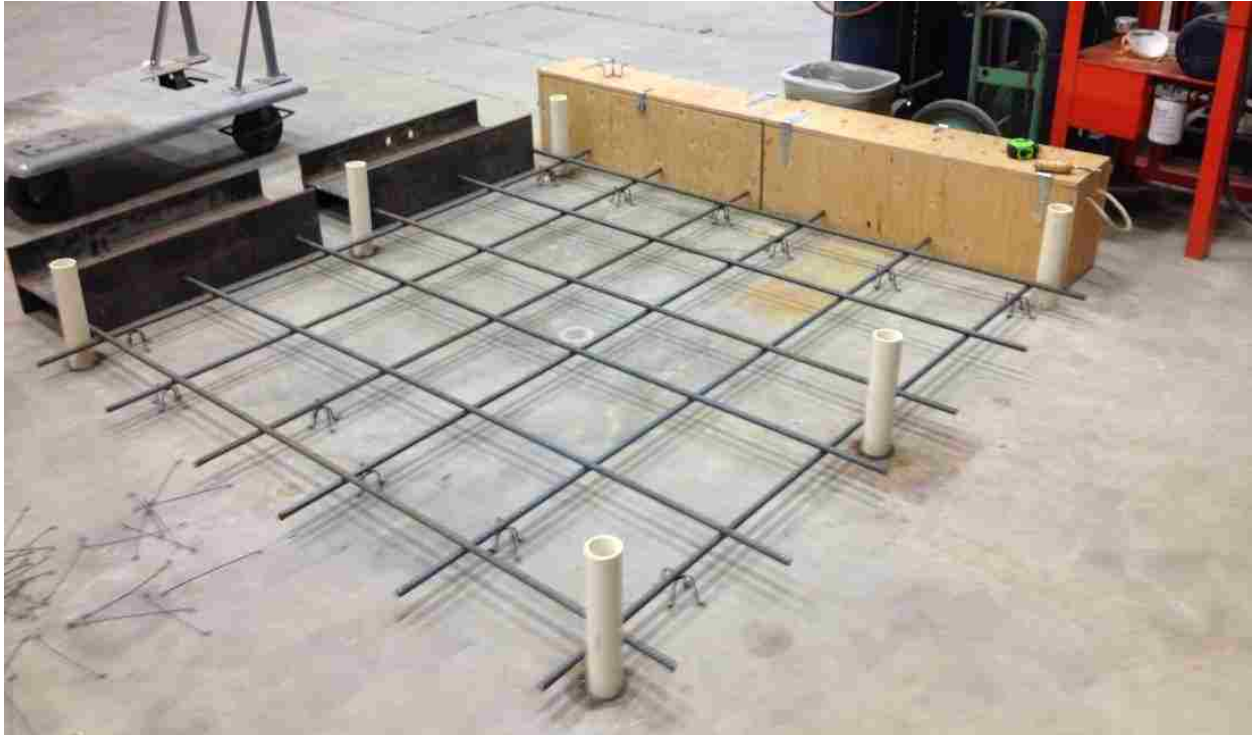
Figure 3-5: Tying the Footing Rebar
